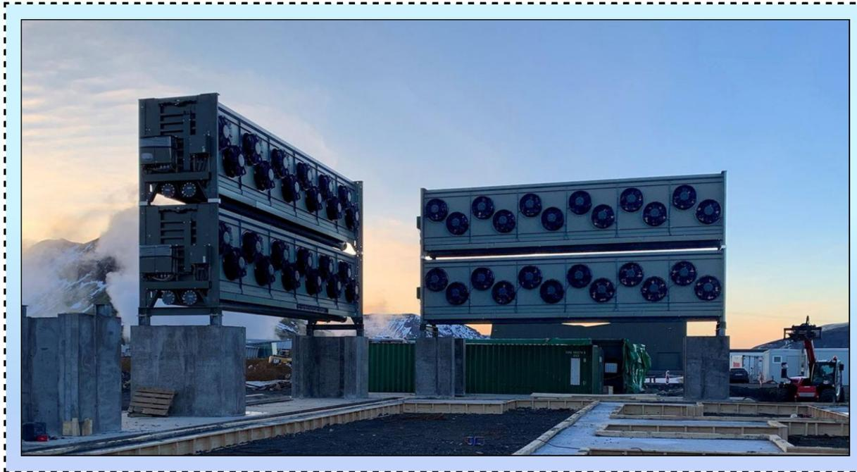
*Climeworks'* high quality direct air capture technology removes CO<sub>2</sub> from the air, after which it is destined for permanent storage underground.
